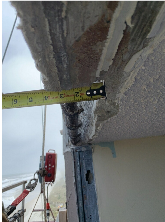
Picture 2: Unit 601 window header repair
