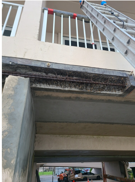
Picture 1: Slab edge repair at Unit 103/104
